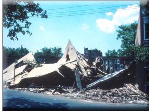
Image 2: In 1980, an FDNY firefighter was killed when a burning three-story, wood-frame structure suddenly collapsed, flattening the adjoining one-story building he was working in.
