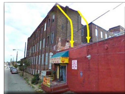
Image 4: Two Philadelphia firefighters were killed when part of a four-story, heavy-timber building collapsed on an adjacent structure, burying the firefighters inside. The yellow arrows indicate the wall that collapsed.
